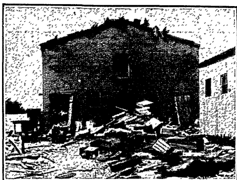
MAIN BUILDING WRECKED BY THE EXPLOSION
