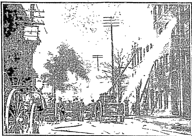
FRONT STREET—SHOWING SIDE OF BURNING BUILDING
