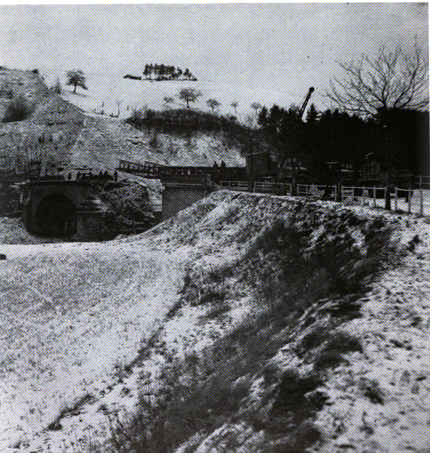
Bridge at Diekrich
