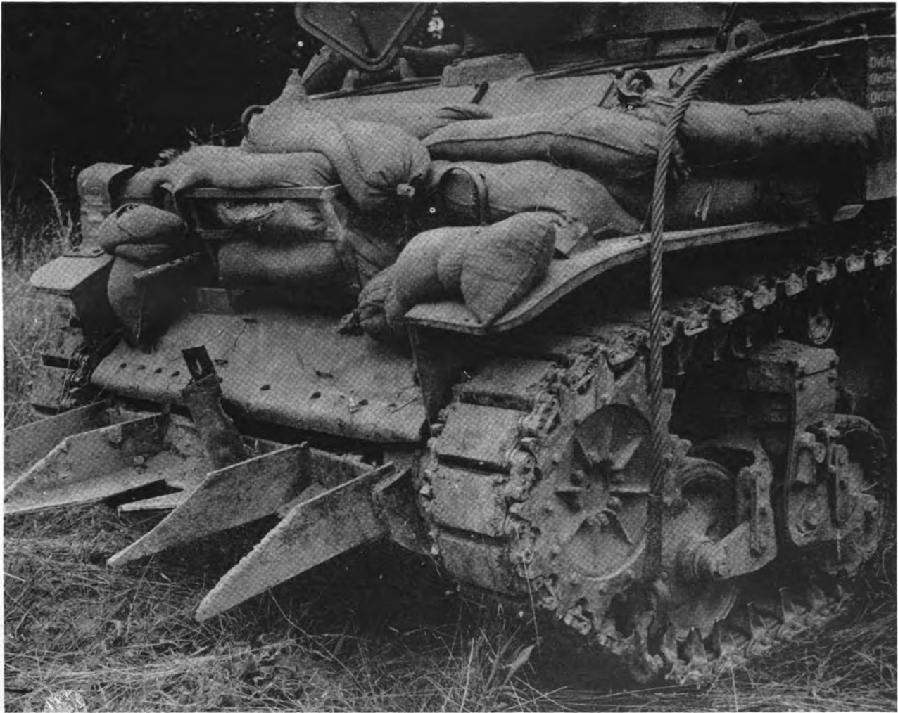
Tank equipped with teeth for making opening in Normandy hedgerows
